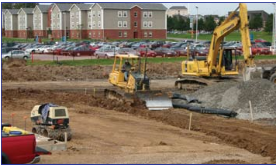
Admar installed the machine control system on DDS's John Deere 700H dozer and provided the training to get DDS personnel comfortable working with the system.
